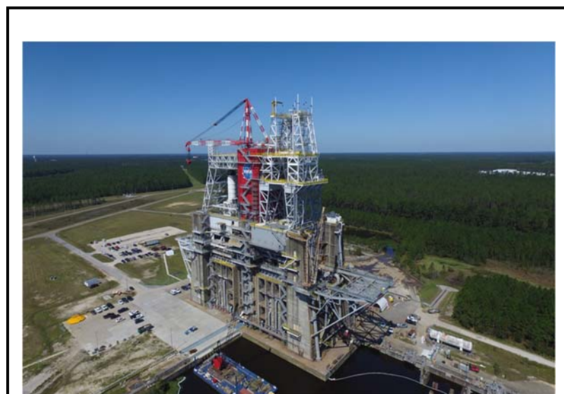
The B2 Test Stand at Stennis Space Center. This South East aspect shows the additional superstructure added to the stand to accommodate the height of the SLS Core Stage, as well as the completed tarmac in front of the stand.
