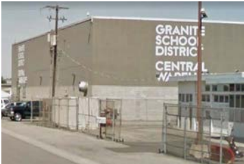
Warehouse 340 West 3050 South
