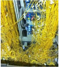
Figure 1 Paper labeling of optical fibers
