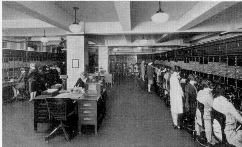
Fig. 8—Private branch exchange—1600 stations, 148 lines to Central Office, 151 tie trunks to other private branch exchanges, 42 switchboard positions, 60 operators and 24 hour service.
