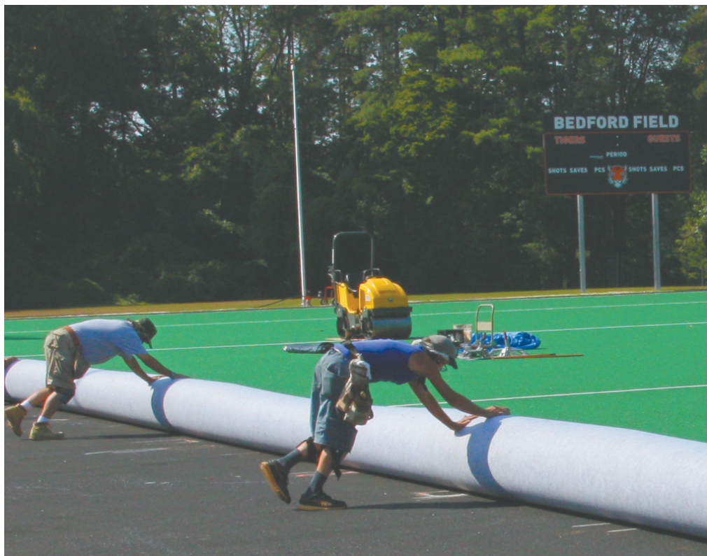
Workers from Play Safe Turf & Track of Ithaca, N.Y., installed artificial turf at Bedford Field this summer. The process involved sewing the turf to the ground in the sections.
