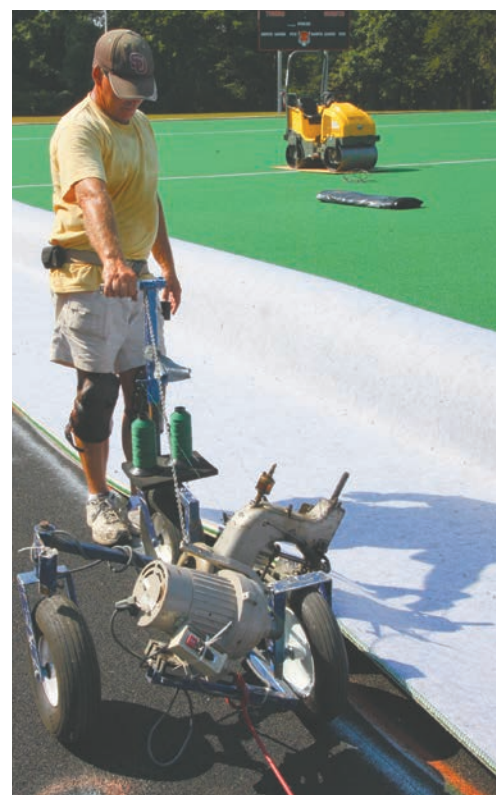
Workers from Play Safe Turf & Track of Ithaca, N.Y., installed artificial turf at Bedford Field this summer. The process involved sewing the turf to the ground in the sections.
