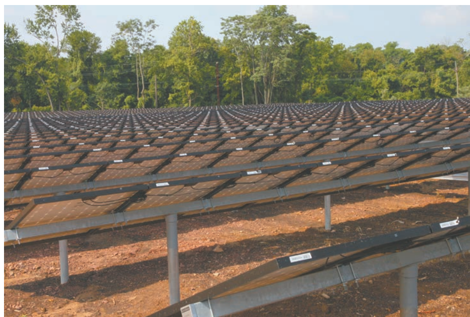
Installation of the University's solar collector field, comprising 16,500 photovoltaic panels across 27 acres in West Windsor, is scheduled to be completed this fall. The system will produce solar power to support the University's annual electrical needs.
