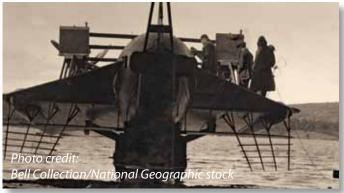
HD-4 out of water on a marine rail showing her elaborate under water foil structure. She was a huge craft of 60 feet in length and weighing 10,000 lbs.
