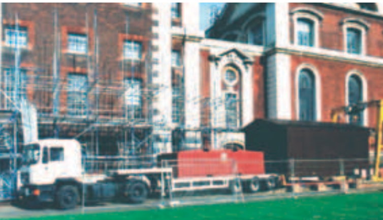
Waste containers outside the King William building
