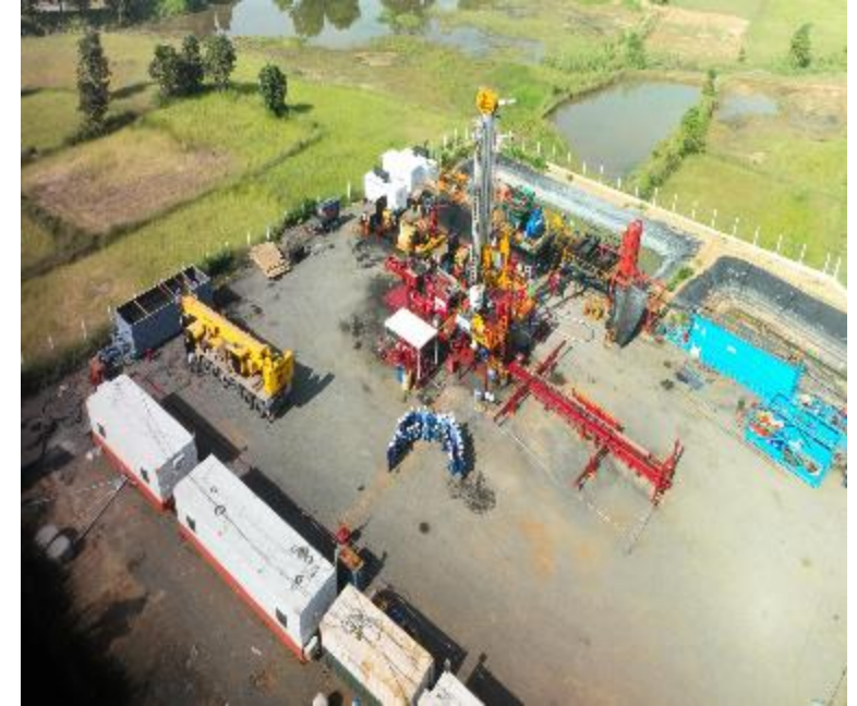
CBM RIG in location
