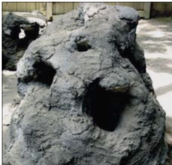
Figure 4. Fish house, constructed using cement and limestone.
