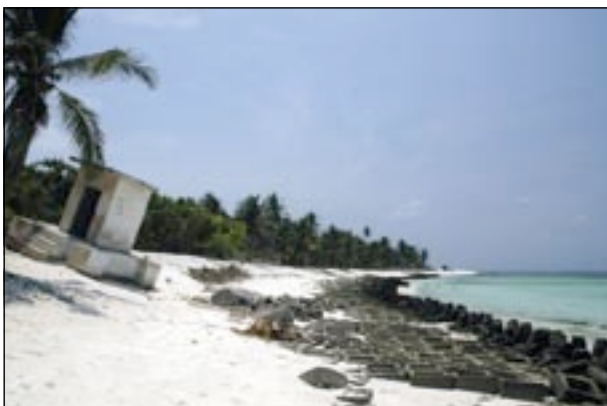
Figure 9. Cement tetrapods and other modules deployed to prevent erosion. A cyclone in 2004 caused significant loss of beach sand and infrastructure damage. Photo: JERKER TAMELANDER.
