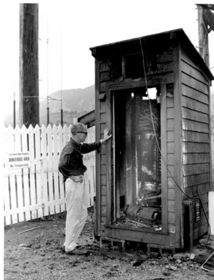
Fig. 14. The experimental WWVB station in Boulder was destroyed by lightning shortly before the Fort Collins station went on the air.
