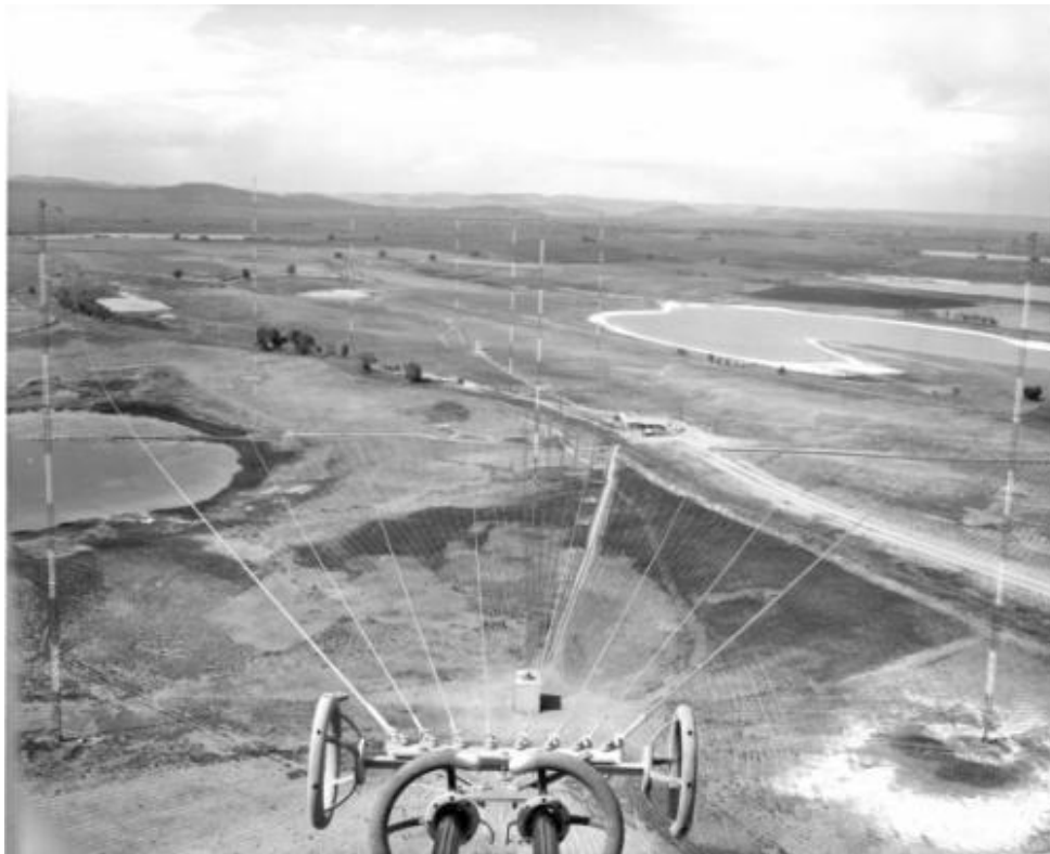
Fig. 12. View of the antenna array from the top of Tower 1.
