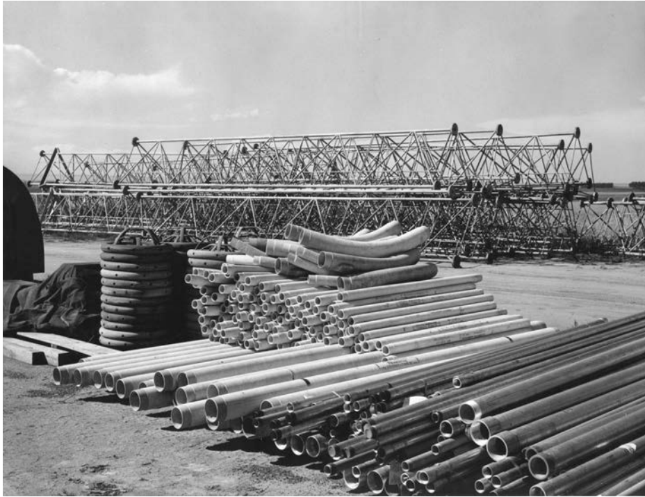
Fig. 11. WWVB antenna parts on the ground prior to assembly, 1962.
