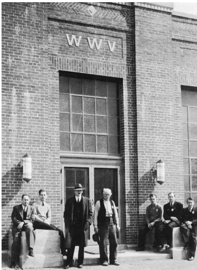
Fig. 2. WWV transmitter building, Beltsville, Maryland, 1943.
