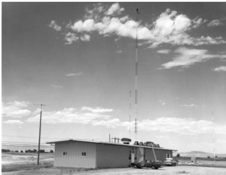
Fig. 13. The original WWVB transmitter building in Fort Collins, completed in July 1963.
