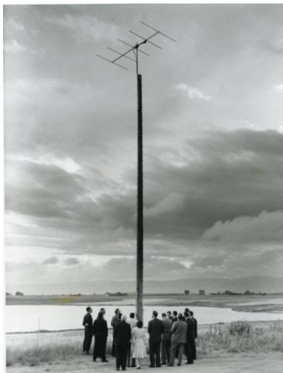
Fig. 18. Antenna used to receive phase corrections from Boulder. Photograph taken at WWVB / WWVL station dedication, August 13, 1963.
