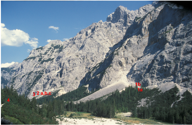
Fig. 1. The 400–600 m high first ascend of the Reintal North Face (N 47°25′; E 11°06′ at the left fringe; E 11°04′ at the right fringe). Rockfall collector positions are indicated by number 1a to 4. Significant intermediate storage is visible on ledges and in couloirs.
