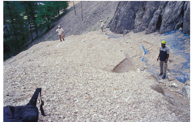
Fig. 3. 56 tons of rockfall (300 kg/m 2 ) on net 1a were deposited on 14 June 2003 from 07:00 p.m. to 08:00 p.m. by a secondary rockfall event in response to a heavy rainstorm. The blue rockfall net is visible on the right-hand side where rockfall deposits had already been removed. The rucksack and the three people indicate the size of the rest of the net, which is still covered by up to one meter of rockfall deposits.
