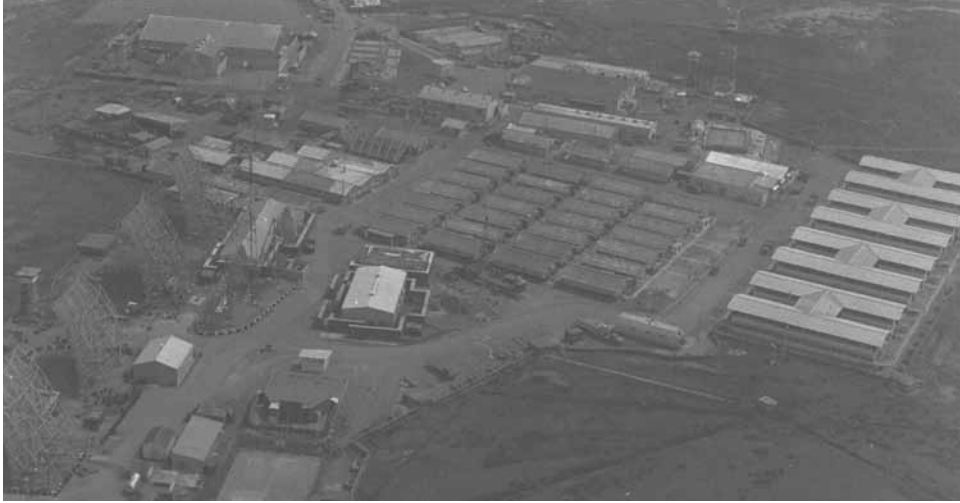
Aerial view of the communications complex at Phu Lam
