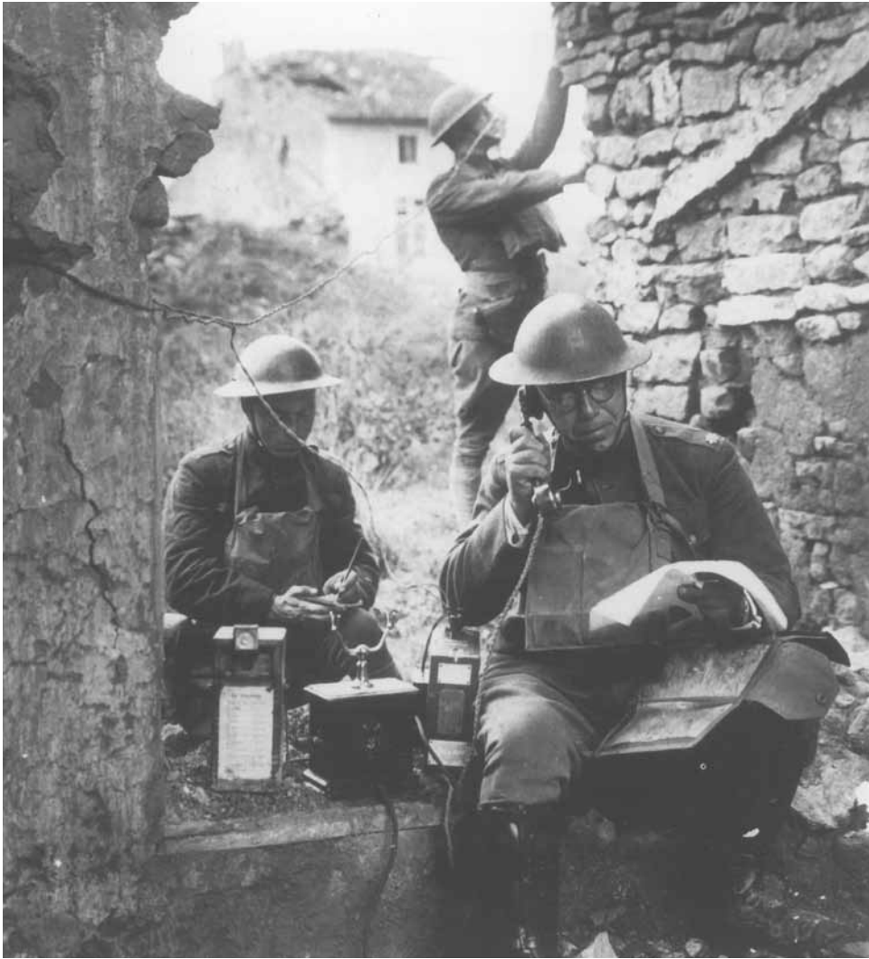
Testing a telephone line left behind by the Germans at St. Mihiel
