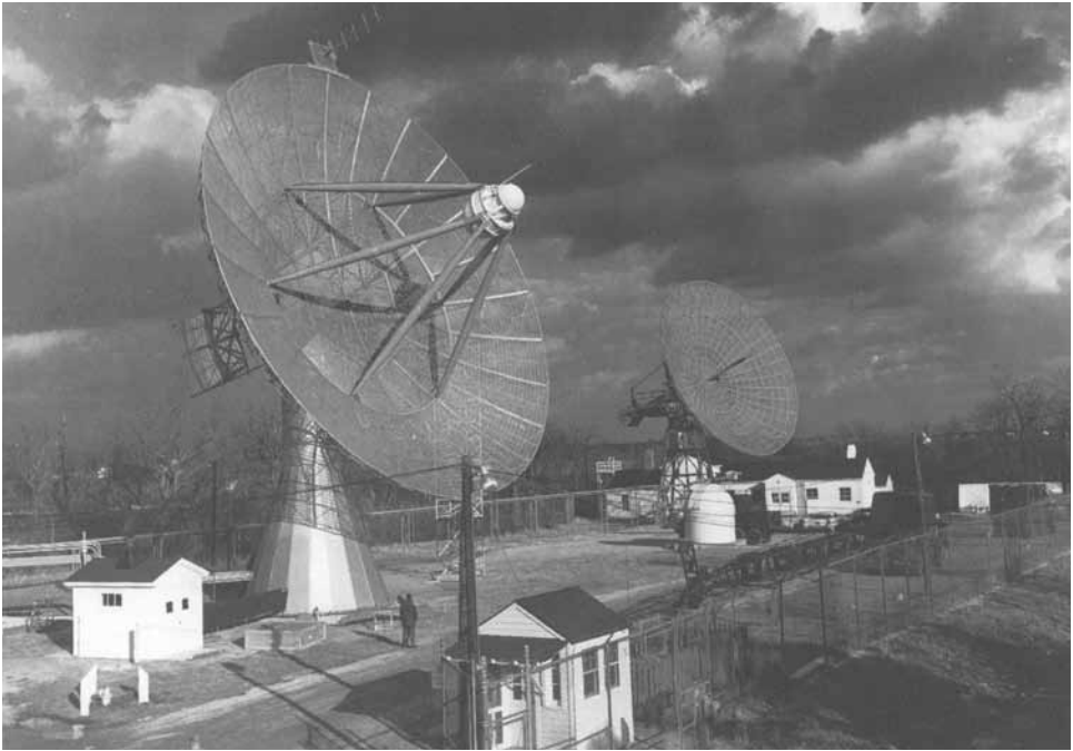
The Signal Corps Engineering Laboratory's astrophysics observatory at Camp Evans, New Jersey, 1959. The parabolic antennas tracked the earliest U.S. and Soviet satellites.
