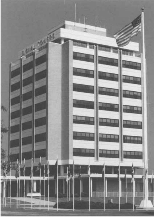
Signal Towers at Fort Gordon, Georgia, the “home of the Signal Corps”
