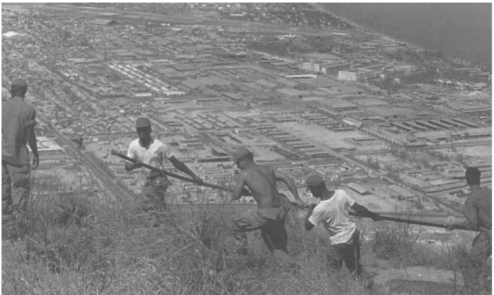
Laying cable on Vung Chua Mountain. Clockwise from left, helicopter delivers 300-pair cable to Company D, 40th Signal Battalion; unreeling the cable; hauling cable down the mountain with the city of Qui Nhon in the background.
