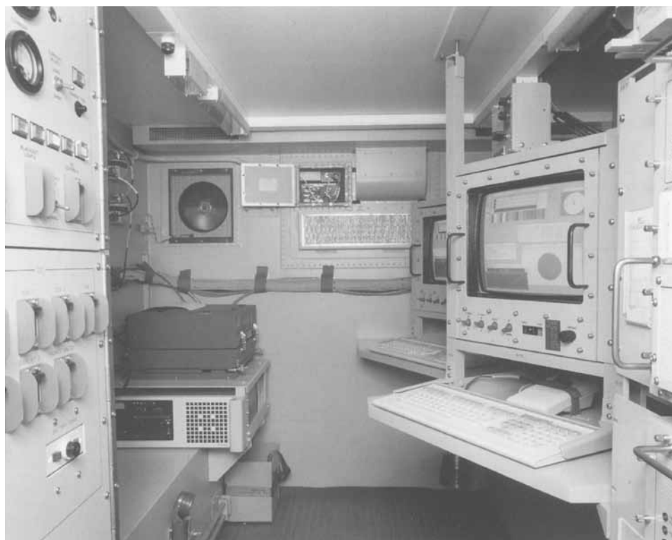
Interior view of shelter housing mobile subscriber equipment
