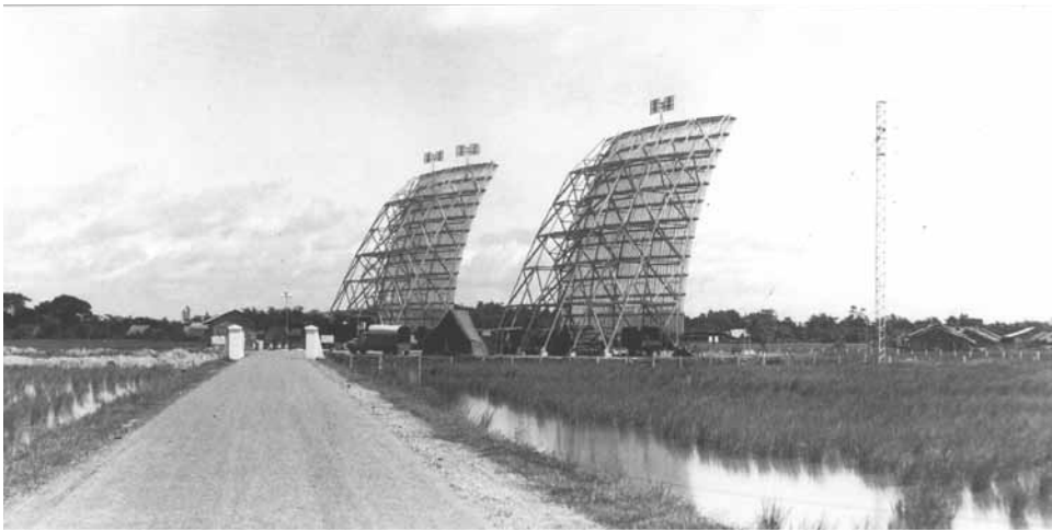
Billboard antennas of the BACKPORCH system at Phu Lam in 1962
