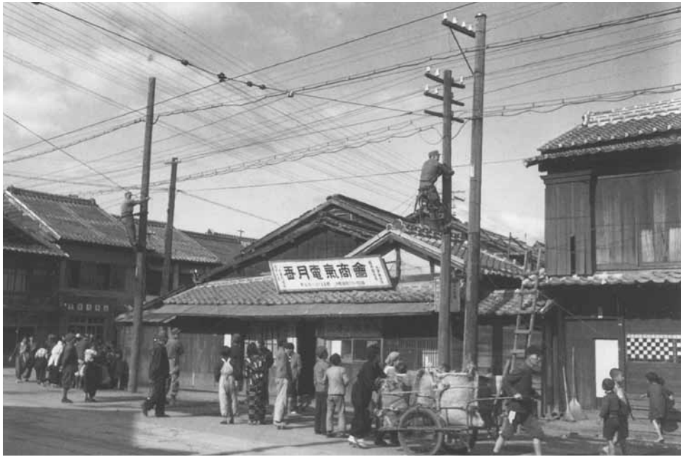
Signal Corps linemen string wire in postwar Japan.
