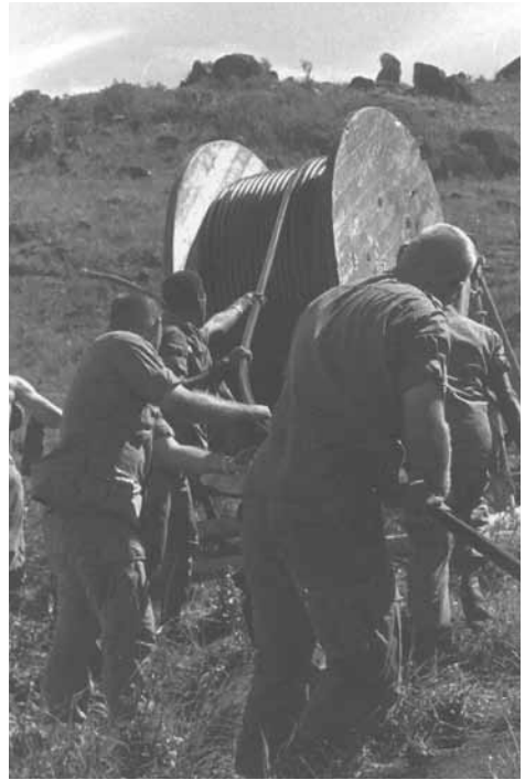
Laying cable on Vung Chua Mountain. Clockwise from left, helicopter delivers 300-pair cable to Company D, 40th Signal Battalion; unreeling the cable; hauling cable down the mountain with the city of Qui Nhon in the background.
