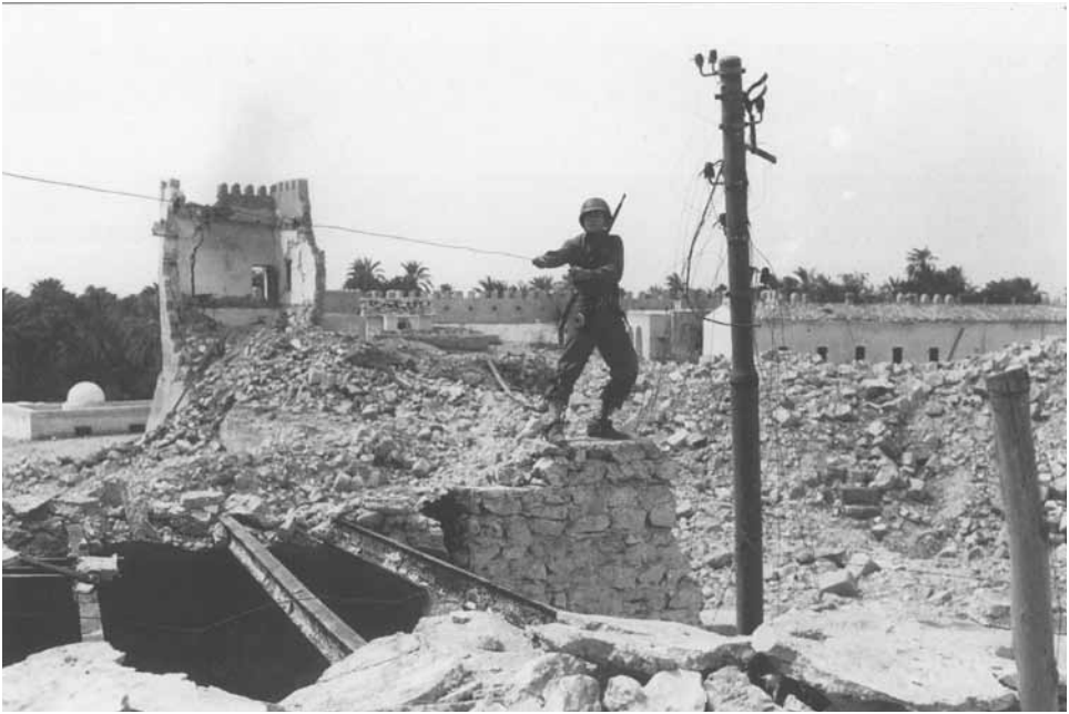
Repairing telephone lines in Tunisia
