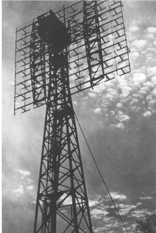
The SCR-271 radar set used to bounce signals off the moon during Project Diana.
