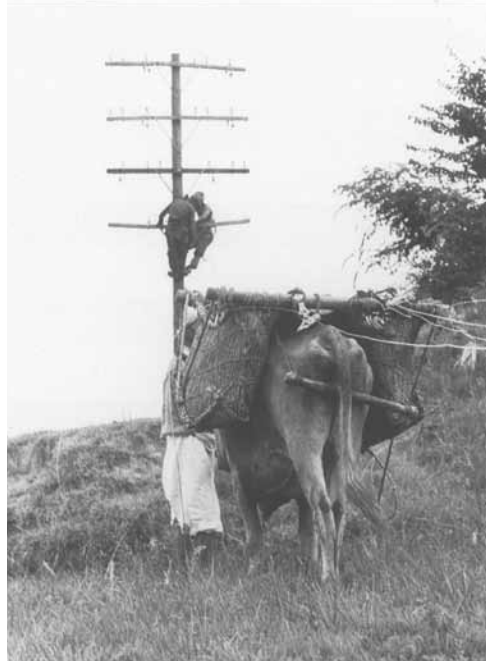
Signalmen in Korea use a water buffalo to stretch wire between poles.
