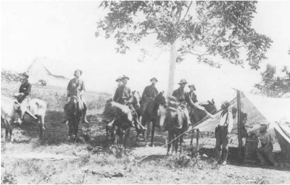
Field Telephone Station No. 4 near San Juan Hill
