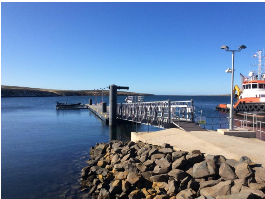
Picture 4 – Small Boat Pontoon with VersaDock.
