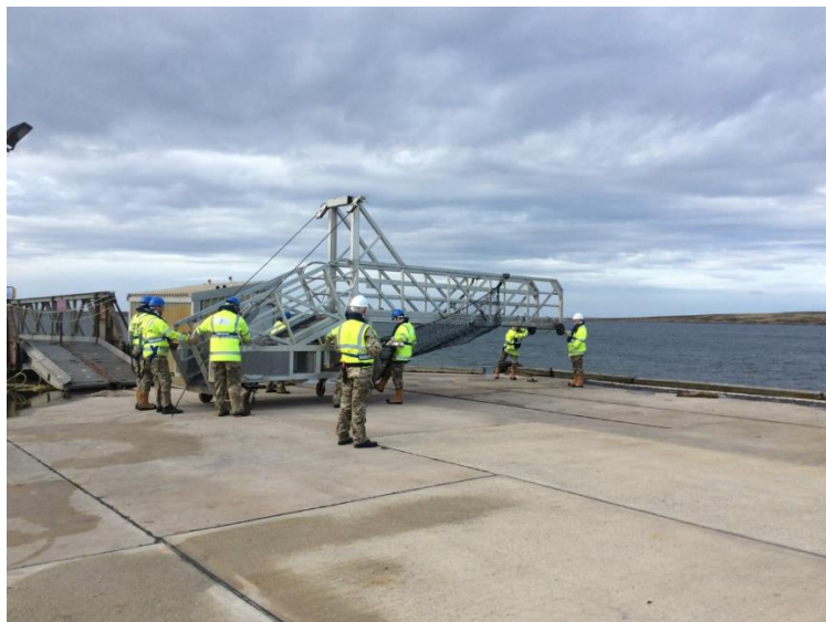
Picture 16 – Cantilever gangway being moved.
