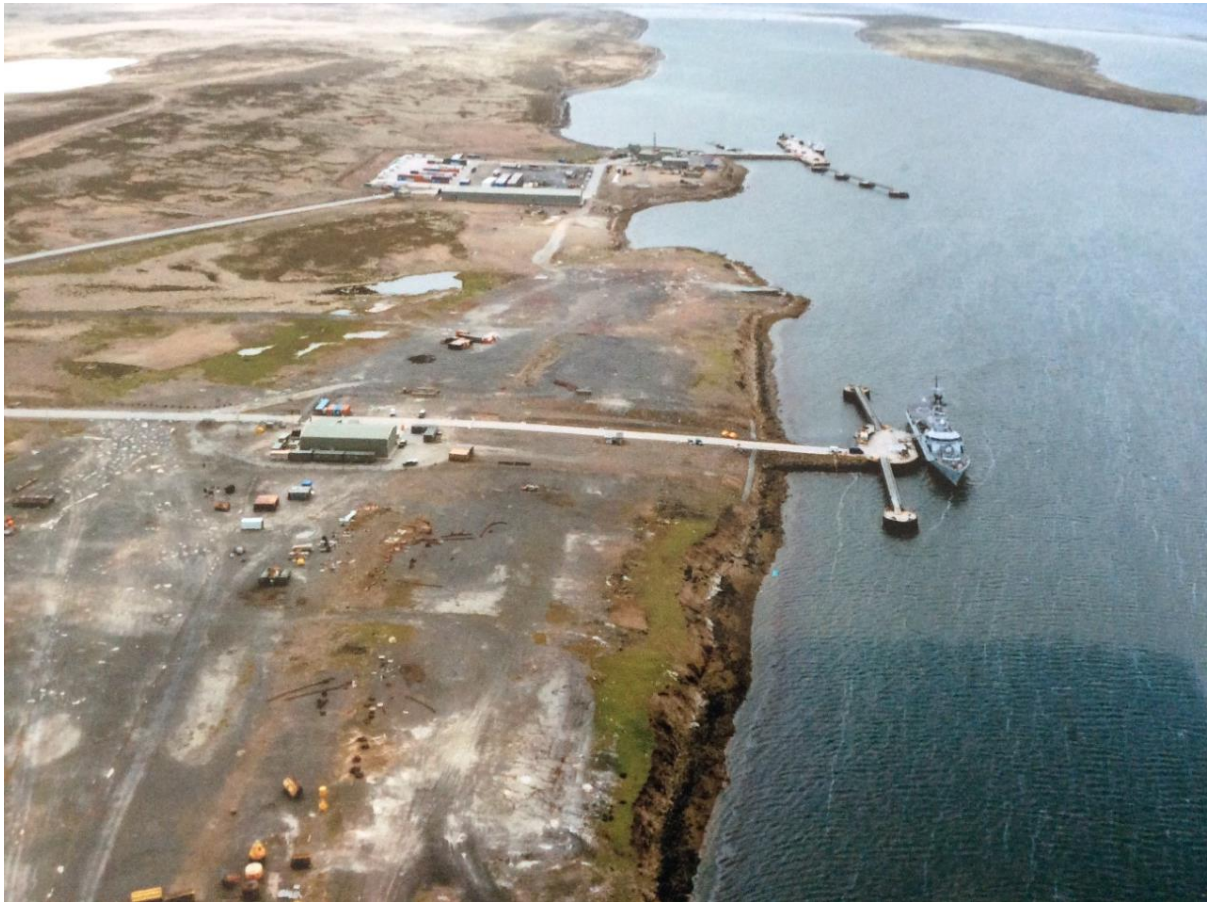
Picture 1 – Aerial view of East Cove Port with West Jetty in the foreground, RoRo Main Jetty in distance.
