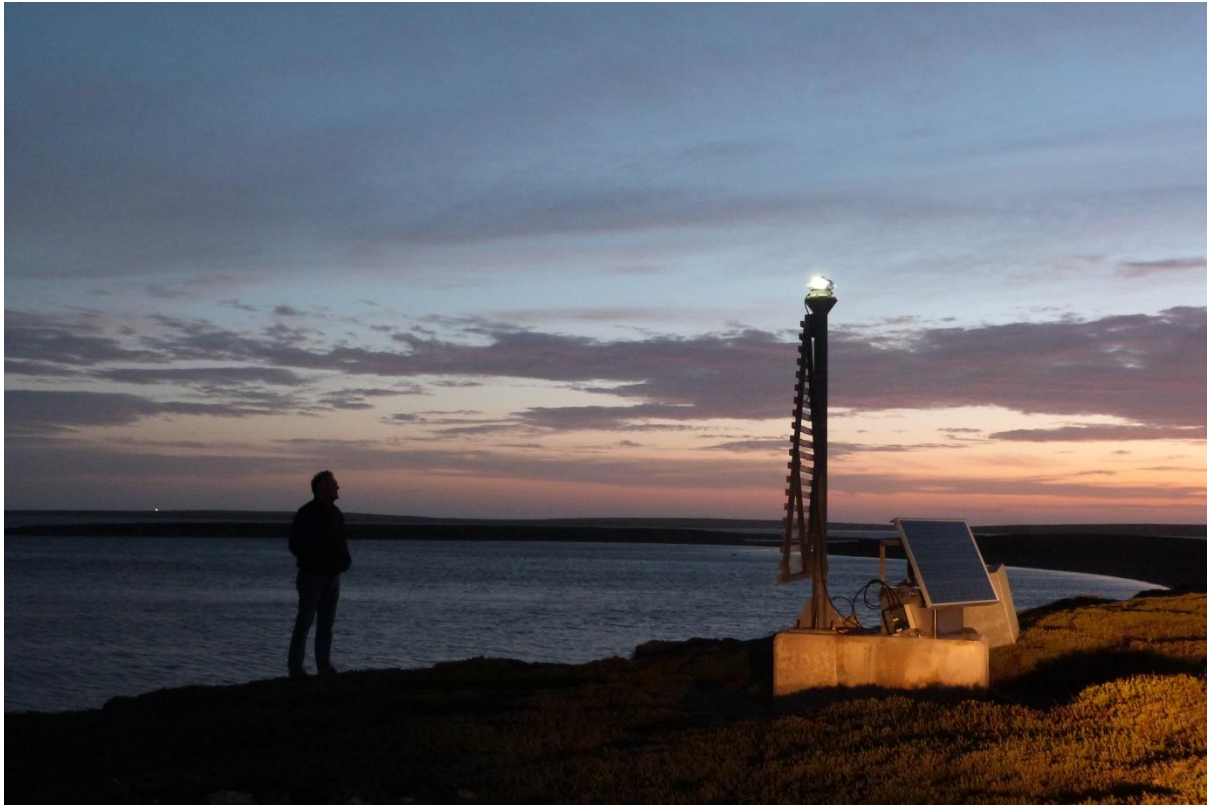
Picture 7 – the newly installed Beacon India.
