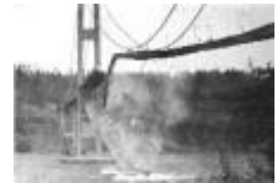
Tacoma Narrows Bridge shaking itself apart because it was too springy and started to resonate in the wind
