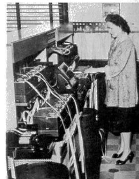
Operator relaying messages with "torn tape" central office equipment
