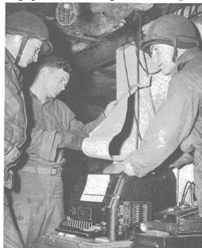
Field headquarters Teletypewriter installation of First Division at Sourbrodt, Belgium, January, 1945
