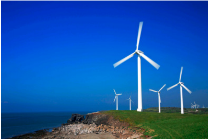
Wind turbine: Synchronized rotor blade control actuators
