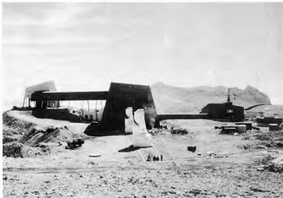
The site of the IRAM interferometers at Plateau de Bure, 120 km south of Grenoble at 2500 m altitude with (from left to right) cable car station, assembly hall or shelters and living quarters. Two steel mounts in foreground on their rail-track.
