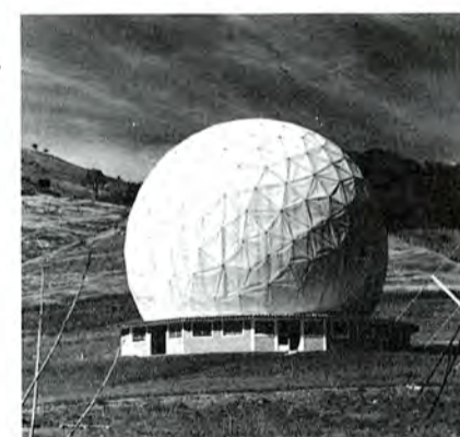
The Itapetinga 13.7-m radio telescope, inside a 23-m radome, for mm-waves, recently installed near the town of Atibaia, São Paulo, Brazil.
