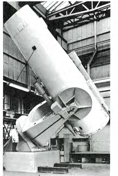
The telescope during construction in the British factory of Sir Howard Grubb Parsons and Company Limited.
