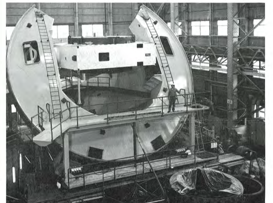
The telescope mount of the 150-inch Anglo-Australian telescope, built by Mitsubishi Electric Corporation, and currently being installed at Siding Spring, New South Wales.
